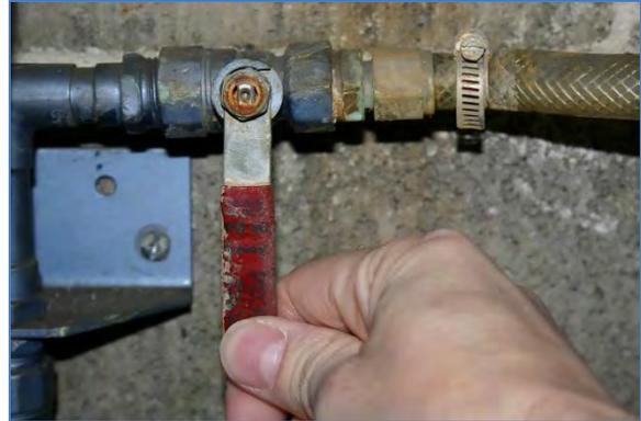
4. Close water supply at shut-off valve.
