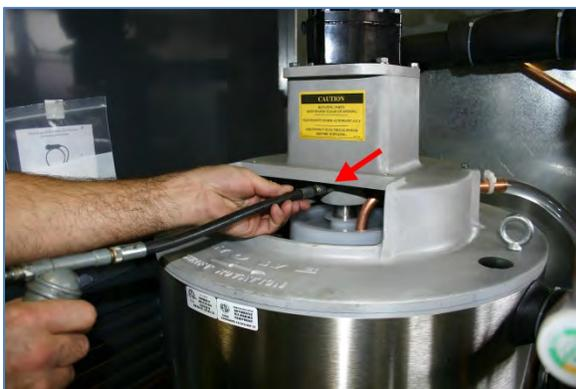
Zerk fittings are installed on both the top and bottom castings as pictured above, for ease of routine maintenance.
