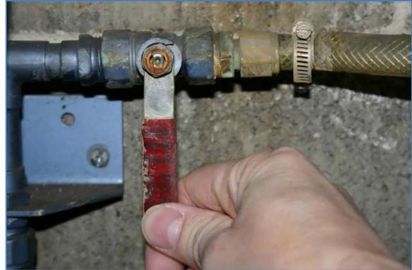
4. Close water supply at shut-off valve.
