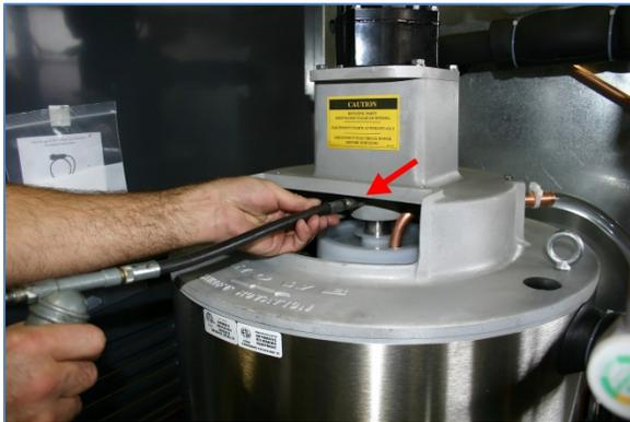
Typically, only one squirt of the grease gun is required or until you feel resistance on the pump.
