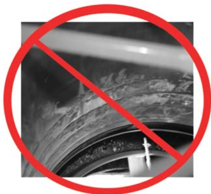
Improperly adjusted TXV
