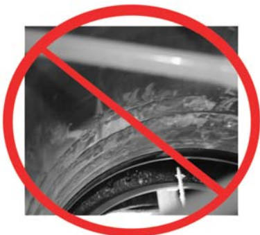
Improperly adjusted TXV
