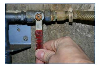
4. Close water supply at shut-off valve.
