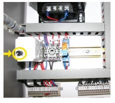
After proper adjustment (referenced on the Quick Step Guide) record off delay timer set point.
